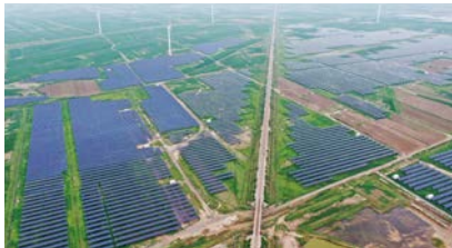
65MW Cangzhou, Hebei, Chine, 2018 Base Top-runner Haixing
